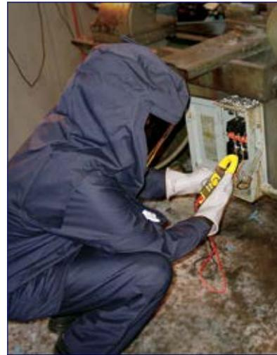
*After operating the disconnect switch, a worker still needs to verify deenergization. Exposure to live parts is inevitable, so PPE is required.*
