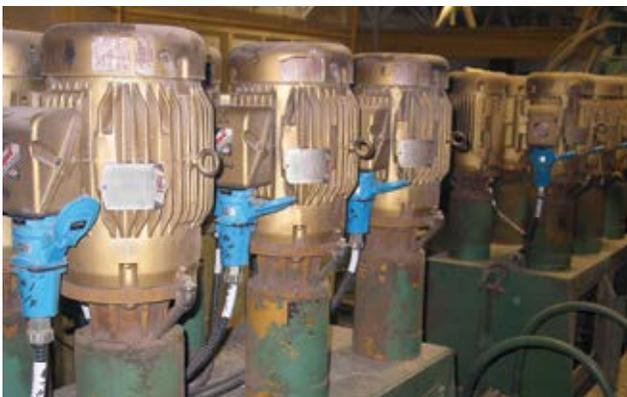
*Decontactors enable quick motor change-outs.*
